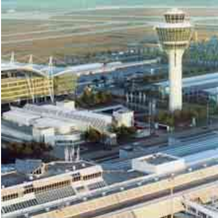
1 Munich Airport Center, Germany
